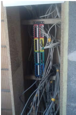
Fig. 4. Patch panel organizing connection of Raspberry Pi computers to sensors.
