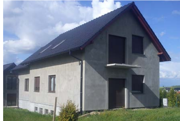
Fig. 2. Experimental building area.
