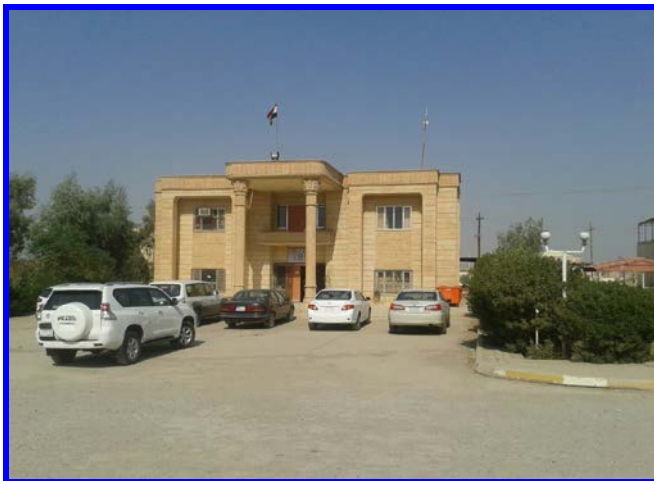
Figure 3: The building of the dean of Kirkuk Technical College
