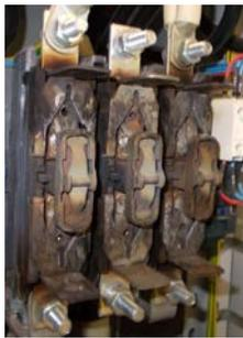
Fig 3. Burned power contacts
