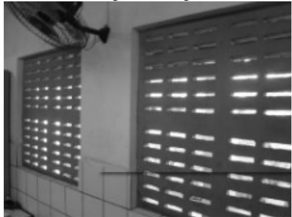
**Figure 3: Walls with holes in a classroom (no thermal insulation)**
